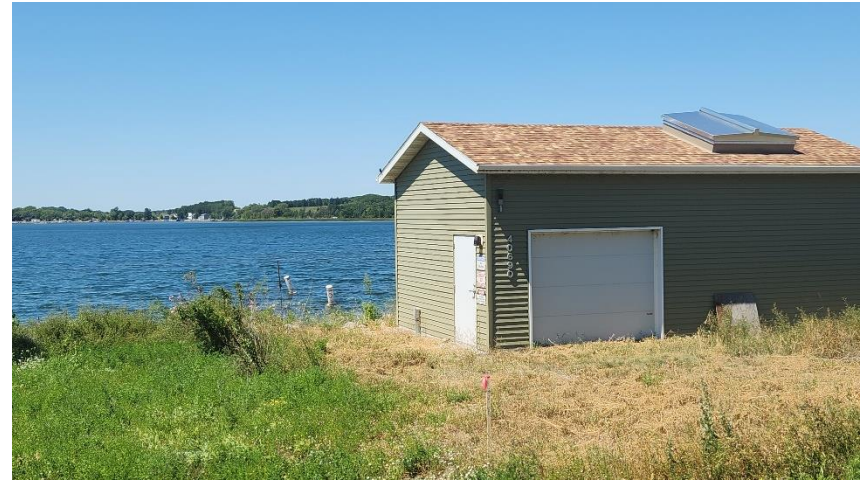
Pump House at Devils Lake Pumping Project, Perham MN.
